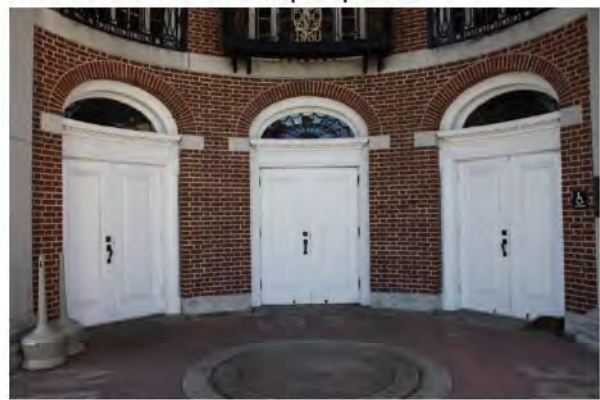
Photo 24: First story entries, northern façade
