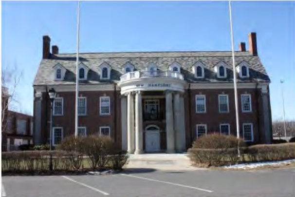
Photo 19: New Hampshire building main northern facade
