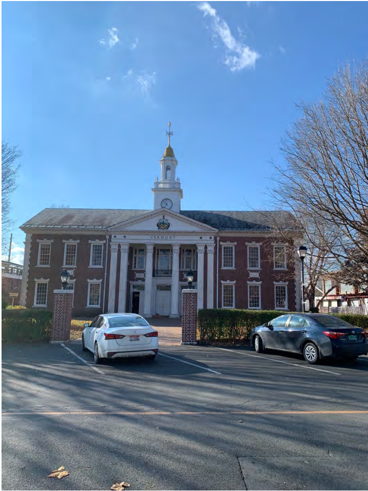
PHOTO OF BUILDING FROM NORTHWEST
