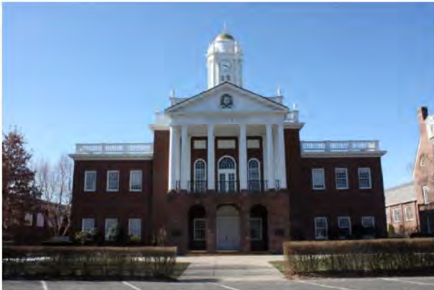
Photo 25: Connecticut building northern main facade
