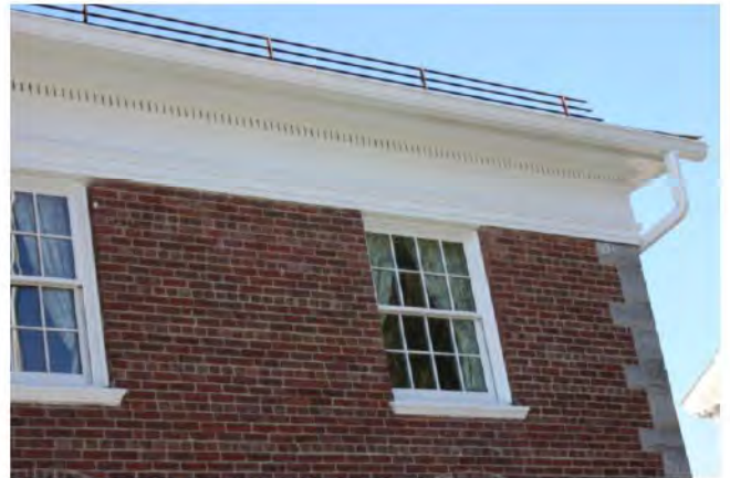
Photo 10: Wall and roof details
