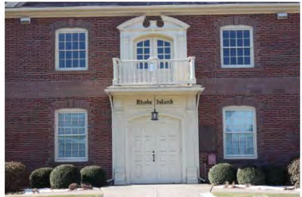
Photo 34: Main entry and balcony, northern facade
