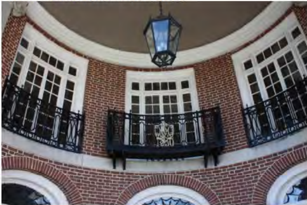
Photo 23: Balconies of round portico
