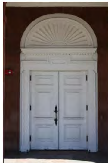
Photo 30: Main entry door, northern facade
