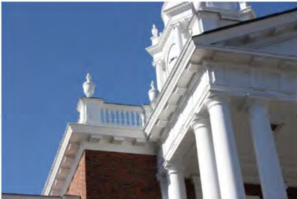
Photo 27: Portico and roof balustrade details
