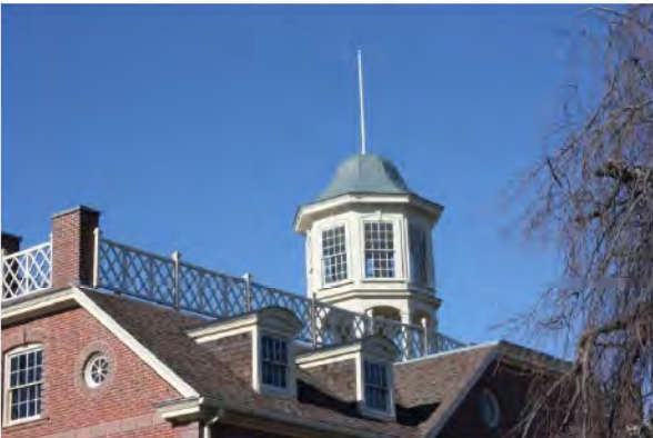
Photo 33: Cupola and rooftop balustrade
