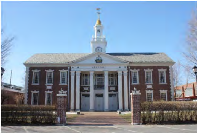
Photo 13: Vermont building main northern facade
